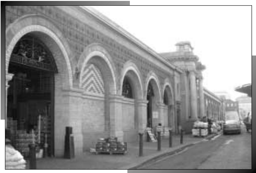
► Markets building, north west inner city.
